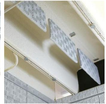
SONEX One Baffles are an ideal solution to reverberation and overall noise problems. These versatile baffles can be used in a variety of settings including: auditoriums, gymnasiums, indoor swimming pools, recreation centers and production facilities. SONEX One Baffles are made from pinta's exclusive willtec® foam, which is Class 1 fire-rated according to ASTM E 84 for flame spread and smoke density. willtec natural also meets the corner burn test UL 1715.
