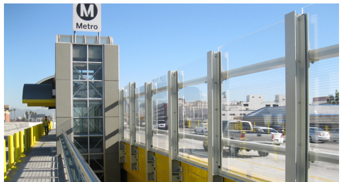
INTERSTATE 110 / 37TH ST BUS STATION - LOS ANGELES, CA
