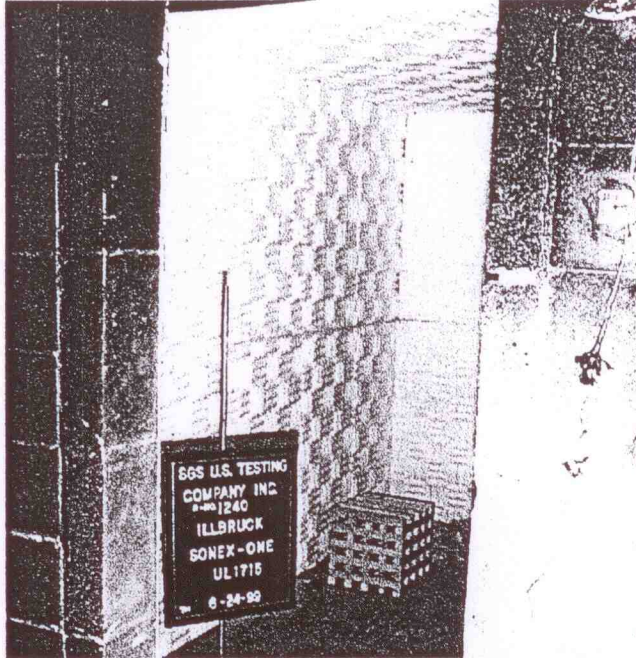
PHOTO 1. Photo of Installation of 'Sonex-One'
