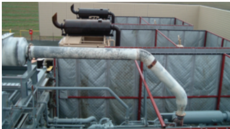
BBC-EXT-R-2" Sound Curtains enclose pumps and compressors.
