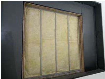
1 #1050R Self-Adhesive Tape, applied to the studs
